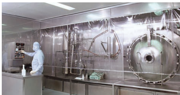
Dedicated collagenase GMP facility
